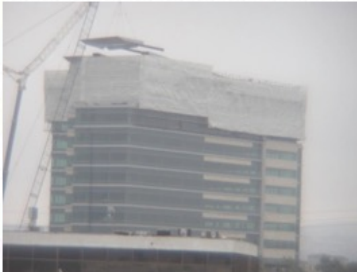
Top two stories being removed
